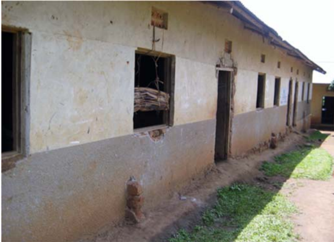
Three Classroom Block before the renovations
